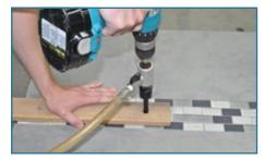
**Step 2** Using a template to stabilize the drill bit, begin slowly drilling with light pressure.
