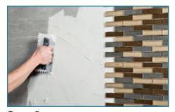
**Step 1** To initiate the bond coat, use the flat side of a trowel and firmly apply thin-set to the substrate.
