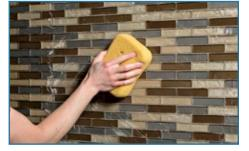
**Step 12** Allow grout to set-up (firm) and smooth finish with a damp sponge. After approximately 2 hours remove grout haze with a lightly damp sponge. For final removal of grout haze, polish with a clean, soft cloth.
