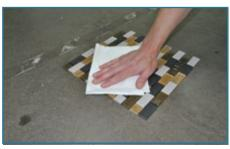
**Step 8** Towel dry the back of the tile and install the sheet as normal.
