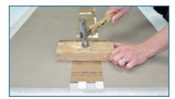
**Step 2** After the installed cement board layer has cured for a minimum of 24 hours, install and grout the tile per the Weave Installation Instructions.
