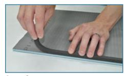
**Step 3** Cut another piece of ¼" cement board to a square size that is larger than a sheet of mosaics. Apply a strip of self-adhesive, compressible, foam weather-strip to one edge of the cement board.
