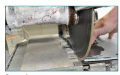
**Step 6** Place downward pressure on the top layer of cement board, turn the saw on and slowly proceed with cutting. The downward pressure should be suffcient to compress the weather-strip, preventing water from fowing under the board, and stabilize the mosaic tiles during cutting.
