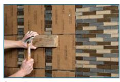
**Step 5** To achieve the flattest possible surface, lightly tap the sheets with a wooden beating block and a finish hammer. To unify sheet transitions, tap from one sheet to the next.
