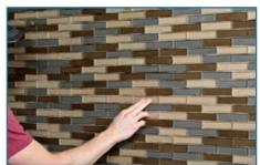
**Step 8** Straighten individual mosaic tiles prior to final set with the goal of creating a consistent overall field of mosaics. To eliminate the sheet pattern, pay particular attention to the transitions between sheets.
