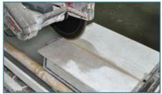
**Step 1** Cover the saw tray with a piece of 1/4" cement board. This will provide a continuous surface that supports the sheet during cutting and prevents mosaic pieces from falling into the tray's cutting channel.
