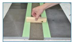
**Step 2** While the bond-coat is still tacky, apply a cement mortar bed (4:1 sand & cement mixture per ANSI A108.1B). Screed the cement mortar bed to the desired substrate depth and cure a minimum of 7 days.
