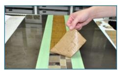
**Step 3** To eliminate voids and visual inconsistencAfter the cement mortar bed has cured a minimum of 7 days, install and grout the tile per the Weave Installation Instructions.
