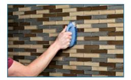
**Step 10** After a full 24 hours (some installations may require extended cure times) use water and a nylon scrub-brush to remove residual glue from the tile. Clean rinse and towel dry.
