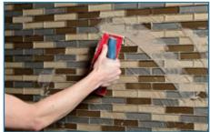
**Step 11** Apply grout with a rubber grout float, forcing grout into joints until full.
