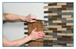
**Step 4** Apply mosaic sheets to the thin-set setting bed, paper side towards you, with light, even pressure. Periodically, check thin-set for skinning (slight drying). If skinning occurs, remove thin-set and reapply.
