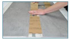
**Step 2** After the build-up layer of thin-set has cured for a minimum of 48 hours, install and grout the tile per the Weave Installation Instructions.
