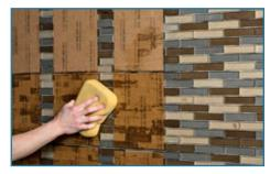
**Step 6** After 15-30 minutes, (floors can be removed sooner) lightly wet the paper. Keep the paper wet by wiping with a damp sponge several times over a 5-10 minute period. After the paper has absorbed the water, the glue will release.
