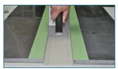
**Step 1** Apply a thin layer (bond-coat) of a recommended thin-set.
