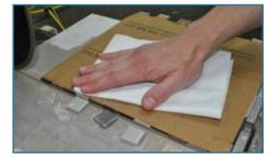
**Step 7** Once cutting is complete, turn the saw off, carefully remove the top layer of cement board and quickly towel dry the mounting paper.
