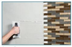
**Step 2** To establish the proper depth of the setting bed, use a 1/4"x1/4" square notch trowel to apply additional thin-set and comb full notches in one direction.
