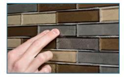
**Step 9** To eliminate voids and visual inconsistencies, push in any translucent glass pieces that have not achieved sufficient thin-set contact.
