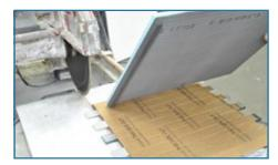
**Step 4** With the saw turned off, place the mosaic sheet, paper side up, on the cement board covered saw tray and align the cut.
