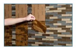
**Step 7** Peel the paper from the tile starting at the corner. Removing the paper while the setting material is still fresh allows for individual tile adjustment and re-inspection of color consistency.
